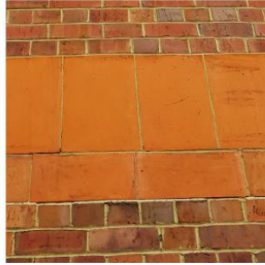
Existing terracotta string course to be reused
