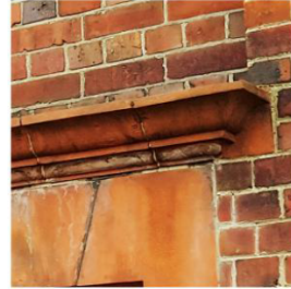
Existing projecting terracotta corbel string course reused
